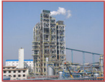
Yueyang Sinopec and Shell coal gasification
