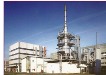
GTL pilot plant Amsterdam
