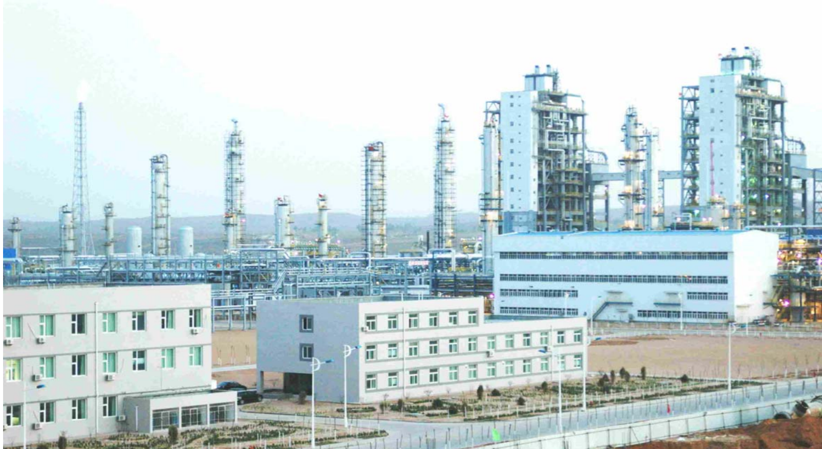
神华鄂尔多斯煤制氢装置-两套壳牌煤气化装置 Erdos DCL H2 unit – Two Trains Shell Coal gasification units
