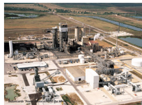
Polk IGCC Power Plant
