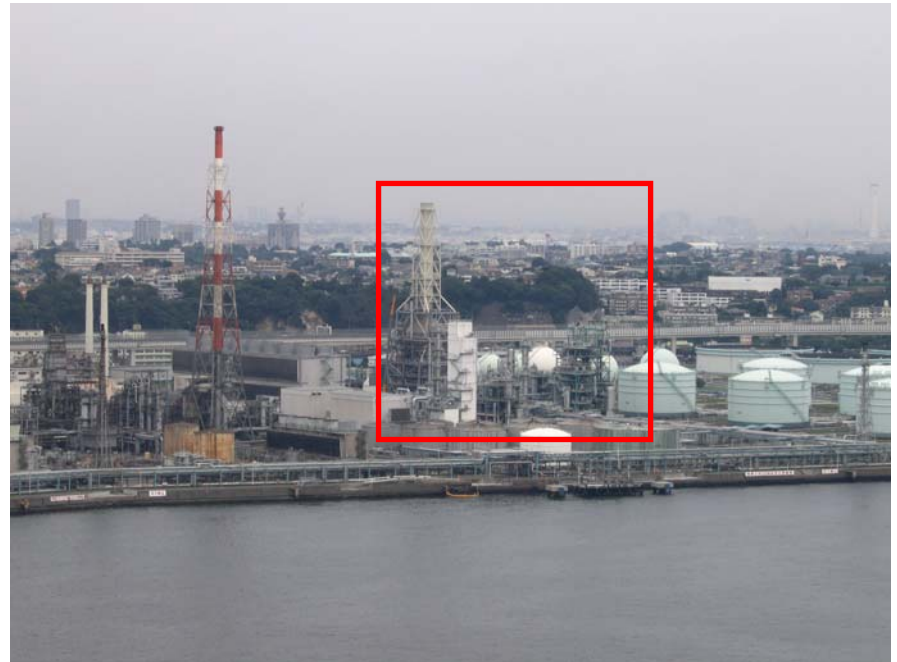
Negishi IGCC, Yokohama, Japan
