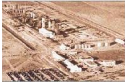
Brownsville, TX 7,000 bpd GTL Plant
