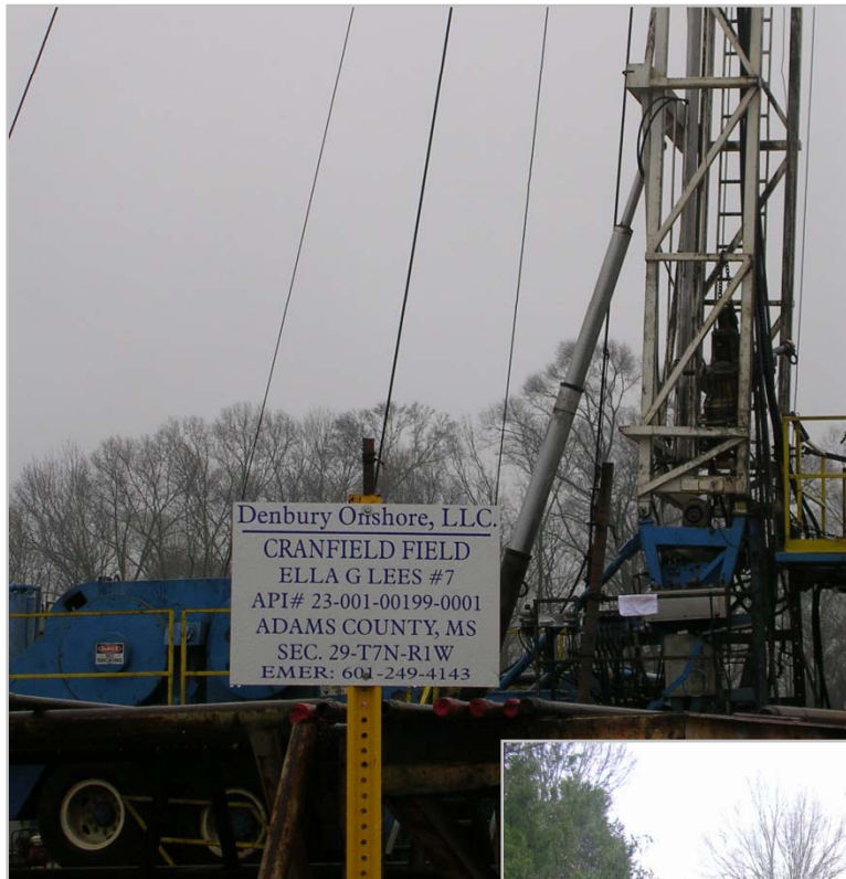
Workover rig on Ella G. Lees #7 Well Phase II Monitoring Well
