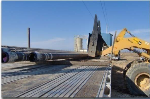
Drill Pipe and Other Infrastructure
